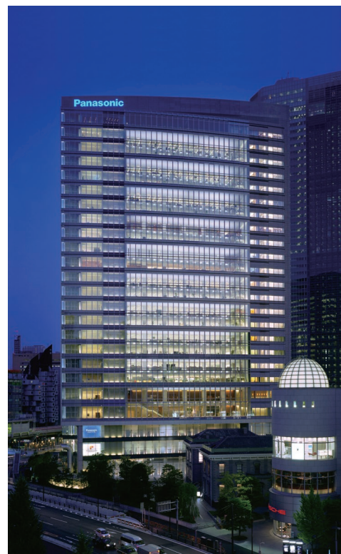
Panasonic Tokyo Shiodome Building (Tokyo, Japan)
